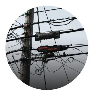
1. This photo from Lafayette Street, Youngstown, OH, shows a severely damaged splice terminal. The terminal's protective case is completely deteriorated, leaving wires exposed to weather and animals. Damaged wires cause service outages.
