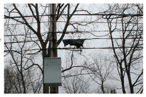
16. This photo from Wexford, Parma, OH, shows a severely damaged splice terminal. The terminal's protective case is missing, leaving wires exposed to weather and animals. Damaged wires cause service outages.
