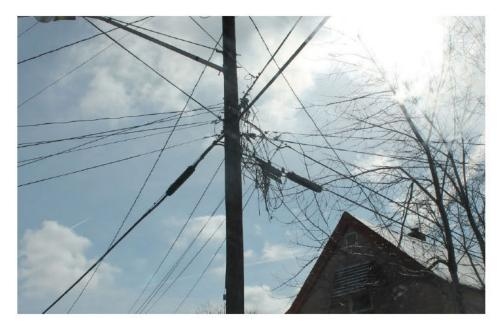
13. This photo from Forest Drive, Pepper Pike, OH, shows an exposed terminal (yellow arrow). The terminal's protective case is hanging open, leaving wires exposed to weather and animals. Damaged wires cause service outages.
