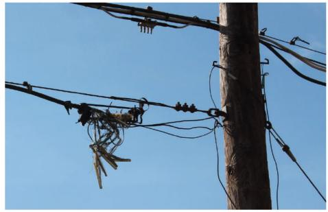
2. This photo from Delaware Avenue, Youngstown, OH, shows a severely damaged splice terminal. The terminal's protective case is hanging open, and the black plastic covering meant to protect wires has fallen off, leaving wires exposed to weather and animals. Damaged wires cause service outages.
