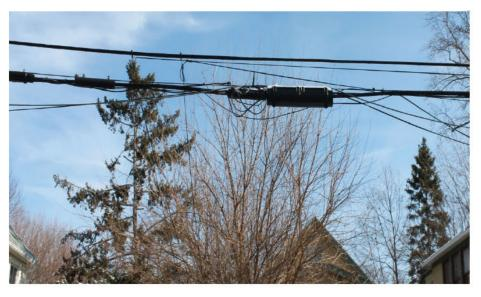
12. This photo from Brown Avenue, Newburgh Heights, OH, shows a severely damaged splice terminal. The terminal's protective case is hanging open, leaving wires exposed to weather and animals. Damaged wires cause service outages.
