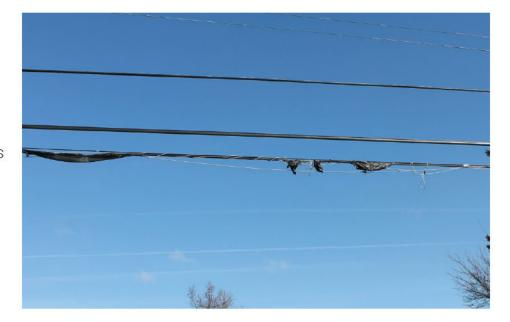
21. This photo from East 2nd Street, Girard, OH, shows a severely damaged splice terminal. The terminal's protective case is hanging open, leaving wires exposed to weather and animals. Damaged wires cause service outages.
