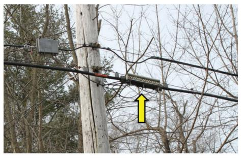
14. This photo from Broadview Road, Seven Hills, OH, shows a disconnected wire hanging above an intersection. The wire is secured to another wire, but the damaged wires are exposed to weather, leading to further degradation of the wire.
