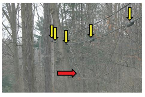
6. This photo from Gates Road, Gates Mills, OH, shows a damaged splice wrapped in a black plastic covering. Once the wrap deteriorates, wires are exposed to weather and animals. Damaged wires cause service outages.
