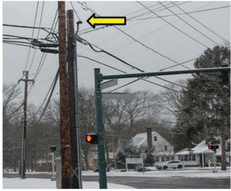
24. This photo from Hillside Street, Cuyahoga Falls, OH, shows a badly damaged cable. Instead of replacing the cable, AT&T installed multiple splice boxes on the cable. Each splice box covers a portion of damaged or defective cable. AT&T also used drop wires to bypass sections of bad cable. Each of the numerous thin wires would have been installed in response to a separate customer complaint.
