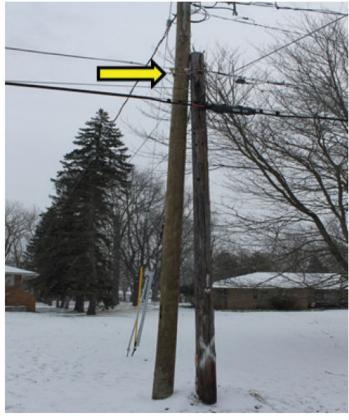
5. This photo from Hillcreek Lane, Gates Mills, OH, shows a badly damaged cable. Instead of replacing the cable, AT&T spliced the cable at least five times on a short strand of cable (yellow arrows). In addition, AT&T used drop wires (red arrow) to bypass sections of bad cable.
