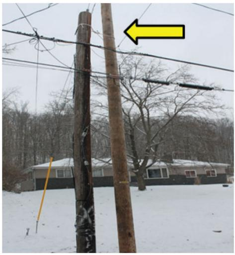
23. This photo from Route 82, Brecksville, OH, shows a double-pole. The old pole (right, with a white spray-painted X) with only AT&T equipment attached to it is tied to the new pole with rope to prevent it from falling (yellow arrow). AT&T has not moved its facilities to the new utility pole. As a result, AT&T's equipment remains connected to old, deteriorating poles, causing potential service and safety concerns.
