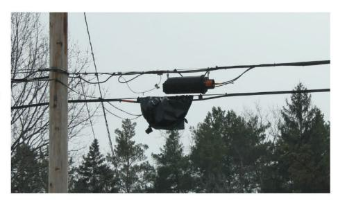
18. This photo from Wolf Lane, Strongsville, OH shows a double-pole. Only AT&T equipment is attached to the old pole (right, with a white spray-painted X). AT&T has not moved its facilities to the new utility pole. As a result, AT&T's equipment remains connected to an old, deteriorating pole, causing potential service and safety concerns. In addition, AT&T's terminal is severely rusted.
