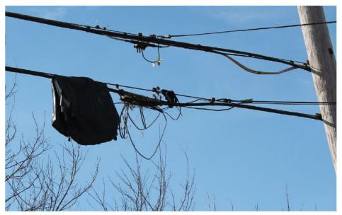
3. This photo from Emery Road, Warrensville Heights, OH, shows unsecured cable. The cable should be secured to the utility pole. The wind blows the unsecured service cable, damaging the copper inside the wire and causing service issues. In addition, this cable is within reach of passersby, causing a public safety hazard.
