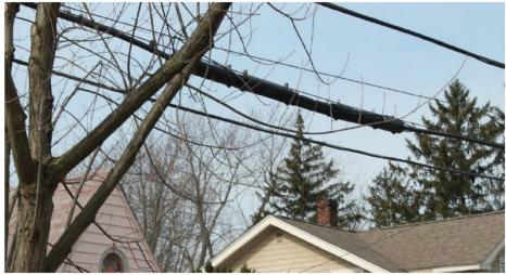
8. This photo from Warrensville Center Road, Maple Heights, OH, shows an unsecured terminal hanging from service wires. The terminal should be secured to the pole. The terminal can fill with water, deteriorating wires and leading to service issues. In addition, a hanging terminal presents a public safety hazard to passersby.
