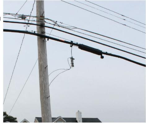
11. This photo from West 48th Street, Cleveland, OH, shows a badly damaged cable. Instead of replacing the cable, AT&T installed multiple splice boxes on the cable. Each splice box covers a portion of damaged or defective cable. AT&T also used thin drop wires to bypass sections of bad cable. Each of the numerous thin wires would have been installed in response to a separate customer complaint.
