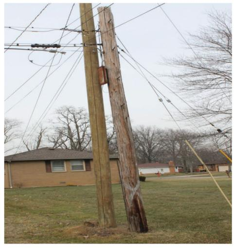
19. This photo from South Thomas Road, Tallmadge Road, OH, shows a hanging pole, or a double-pole that has been cut before AT&T moved its facilities to the new pole. The old utility pole was cut with AT&T's terminal still attached to it. Left dangling, the old pole strains the cables and endangers the public. It is a service, worker, and public safety concern.
