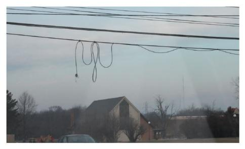
15. This photo from York Road, North Royalton, OH, shows a damaged splice wrapped in a black plastic covering. Once the wrap deteriorates, wires are exposed to weather and animals. Damaged wires cause service outages.
