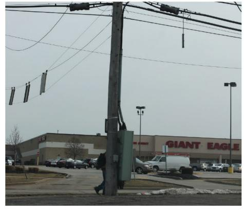
9. This photo from East 135th Street, Garfield Heights, OH, shows a severely damaged splice box. The box's protective case has deteriorated, leaving wires exposed to weather and animals. Damaged wires cause service outages.
