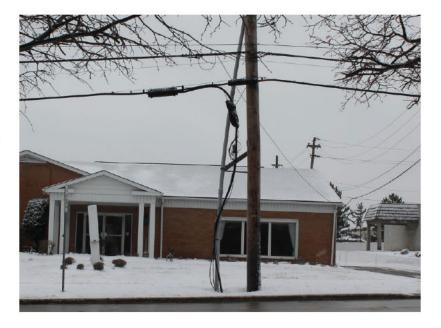
4. This photo from North Linden Lane, Parma, OH, shows a double-pole. The old pole (right, with a white spray-painted X) with only AT&T equipment attached to it is tied to the new pole with rope (yellow arrow) to prevent it from falling. AT&T has not moved its facilities to the new utility pole. As a result, AT&T's equipment remains connected to an old, deteriorating pole, causing potential service and safety concerns.
