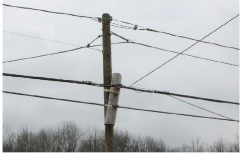
20. This photo from West 2nd Street, Girard, OH, shows a severely damaged cable. Some remnants of a black plastic cover remain. The cable is damaged, leaving wires exposed to weather and animals. Damaged wires cause service outages.
