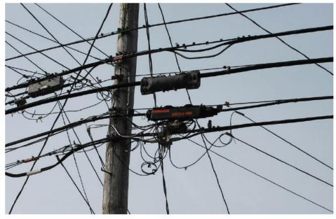
This photo from Evelyn Drive, Seven Hills, OH, shows an unsecured terminal hanging from service wires. The terminal should be secured to the pole. The terminal can fill with water, deteriorating wires and leading to service issues. In addition, a hanging terminal presents a public safety hazard.
