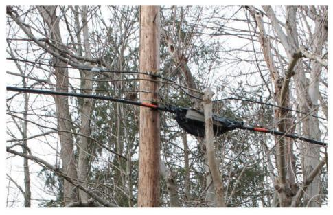
7. This photo from Charles Street, Maple Heights, OH, shows a badly damaged cable. Instead of replacing the cable, AT&T attempted to resolve the problem with multiple slices in a span of a few feet on the cable. Each splice box covers a portion of damaged or defective cable.
