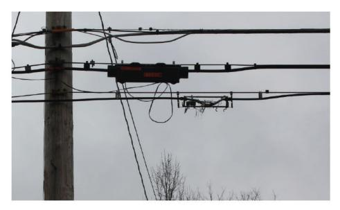
17. This photo from Emery Road, Chagrin Falls, OH, shows a damaged splice wrapped in a black plastic covering. Once the wrap deteriorates, wires are exposed to weather and animals. Damaged wires cause service outages.
