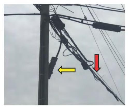
6. This photo from South Belsay Road, Burton, MI, shows a damaged pedestal. Its protective cover is damaged, leaving wires exposed to damage from weather and animals. Damaged wires cause service outages. In addition, the exposed wires are a public safety hazard.
