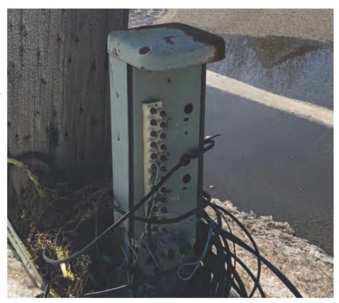
10. This photo from Seymour Road, Flint, MI, shows a rotting pole. AT&T's equipment is the only equipment that remains. AT&T has not moved its facilities to a new utility pole. As a result, AT&T's equipment remains connected to an old, deteriorating pole, causing potential service and safety concerns.
