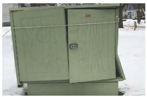
2. This photo from East Main Street, Flushing, MI, shows a damaged pedestal. Its protective cover is damaged, leaving wires exposed to damage from weather and animals. Damaged wires cause service outages. In addition, the exposed wires are a public safety hazard.
