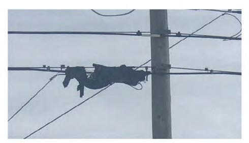
9. This photo from Alpine Avenue, Grand Rapids, MI, shows a severely damaged pedestal. Its protective cover is missing, leaving wires exposed to damage from weather and animals. Damaged wires cause service outages. In addition, exposed wires are a public safety hazard.
