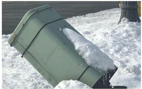
3. This photo from South Main Street, Lapeer, MI, shows a damaged cross-connect box. Instead of replacing the box, AT&T covered it with a black plastic cover. This cover will fall off or deteriorate, leaving wires exposed to weather and animals. Damaged wires cause service outages. In addition, the exposed wires are a public safety hazard.
