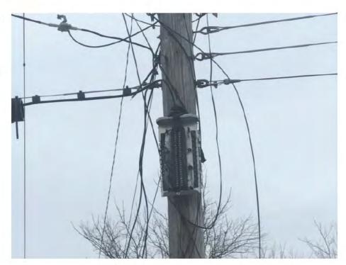
12. This photo from Miller Road, Flint, MI, shows a severely damaged pedestal. Its protective cover is missing, leaving wires exposed to damage from weather and animals. Damaged wires cause service outages. In addition, exposed wires are a public safety hazard.
