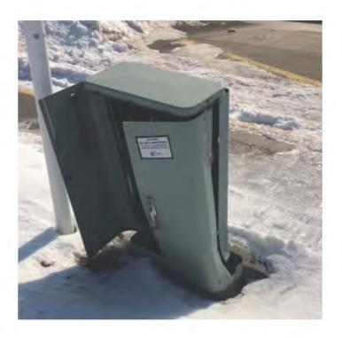
5. This photo from South Lapeer Road, Oxford, MI, shows an unsecured splice terminal and damaged cable. The terminal should be secured to cable, not left hanging (yellow arrow). And cable should be should be secured to the utility pole (yellow arrow). In addition, AT&T used drop wires (red arrow) to bypass sections of bad cable.
