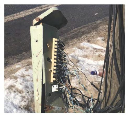
8. This photo from Elms Road, Flint, MI, shows a severely damaged splice terminal. The terminal's protective case is hanging open, and the black plastic covering meant to protect wires has deteriorated, leaving wires exposed to weather and animals. Damaged wires cause service outages.
