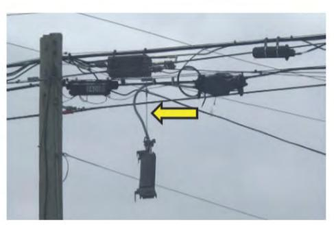
16. This photo from Dixie Highway, Birch Run, MI, shows a severely damaged pedestal. Its protective cover is missing, leaving wires exposed to damage from weather and animals. Damaged wires cause service outages. In addition, exposed wires are a public safety hazard.
