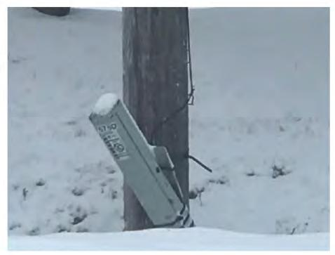
15. This photo from Dixie Highway, Clarkston, MI, shows an unsecured load pot hanging from a cable. Load pots weigh hundreds of pounds and should be secured to the pole. This load pot appears to be supported by a rope (yellow arrow). An unsecured load pot is a safety risk and will result in service issues.
