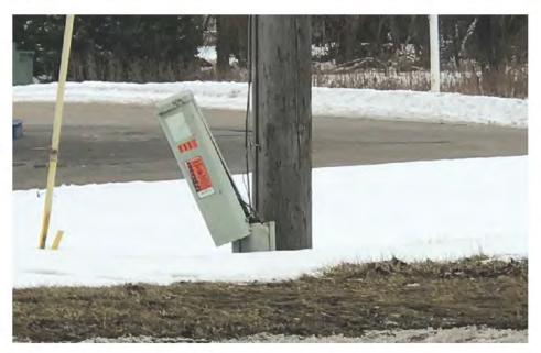
7. This photo from Alpine Avenue, Grand Rapids, MI, shows a severely damaged pedestal. Its protective cover is missing, leaving wires exposed to damage from weather and animals. Damaged wires cause service outages. In addition, exposed wires are a public safety hazard.
