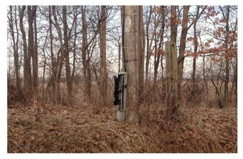
19. This photo from Bloomington, IN, shows an unsecured terminal. The terminal should be secured to the pole, not tied to the cable. The terminal can fill with water, deteriorating wires and leading to service issues. In addition, the terminal is wrapped shut with electrical tape, which is not designed to keep a terminal shut. This presents a serious public safety hazard.
