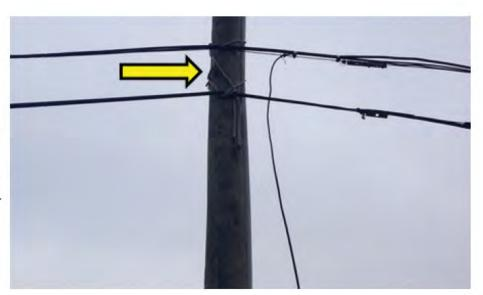
12. This photo from East SR 46, Bloomington, IN, shows a hanging pole, or a double-pole that has been cut before AT&T moved its facilities to the new pole. The old utility pole was cut with AT&T's terminal and cables still attached to it. Left dangling, the old pole strains the cables and endangers the public. It is a service, worker, and public safety concern.
