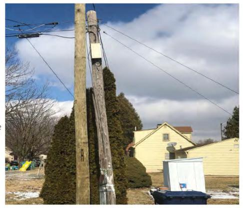
3. This photo from M Street, Bedford, IN, shows an unsecured terminal. The terminal should be secured to the pole, not tied to the cable. The terminal can fill with water, deteriorating wires and leading to service issues. In addition, the terminal is wrapped shut with electrical tape, which is not designed to keep a terminal closed. This presents a serious public safety hazard.
