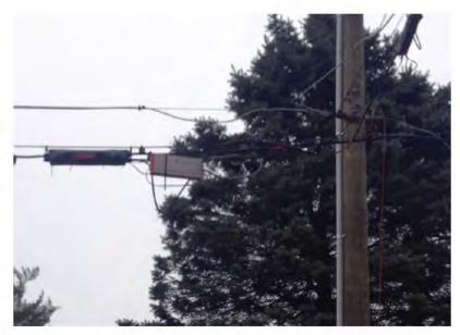
4. This photo from West 32nd Street, Marion, IN, shows unsecured cables. The cables should be secured to the utility pole. The wind blows the unsecured service cables, damaging the copper inside the wire and causing service issues. In addition, these cables are within reach of passersby, causing a public safety hazard.
