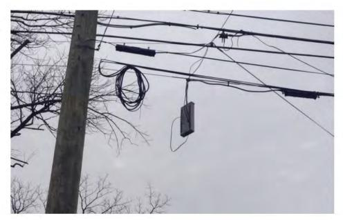
6. This photo from Helmsburg Road, Nashville, IN, shows a double-pole. The old pole (right) is significantly damaged and leaning, putting strain on AT&T's cables and equipment, which remain attached.
