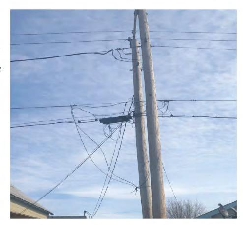
14. This photo from Boone Hollow Road, Bedford, IN, shows a double-pole. The old pole (left) with only AT&T equipment attached to it is tied to the new pole to prevent it from falling. AT&T has not moved its facilities to the new utility pole. As a result, AT&T's equipment remains connected to an old, deteriorating pole, causing potential service and safety concerns.
