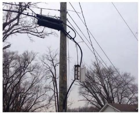
23. This photo from Tunnelton Road, Nashville, IN, shows improperly secured wires. The wires are tied around the utility pole. They will eventually deteriorate, leaving the wires unsecured. The wind blows the unsecured wires, damaging the copper inside the wire and causing service issues.
