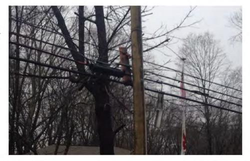
13. This photo from Jefferson Street, Anderson, IN, shows improperly secured wires. The wires are tied around the utility pole. They will eventually deteriorate, leaving the wires unsecured. The wind blows the unsecured wires, damaging the copper inside the wire and causing service issues.
