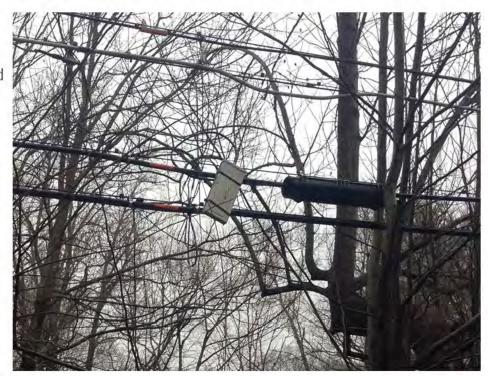
20. This photo from Bloomington, IN, shows an unsecured terminal hanging from service wires. The terminal should be secured to the pole. The terminal can fill with water, deteriorating wires and leading to service issues. In addition, a hanging terminal presents a public safety hazard.
