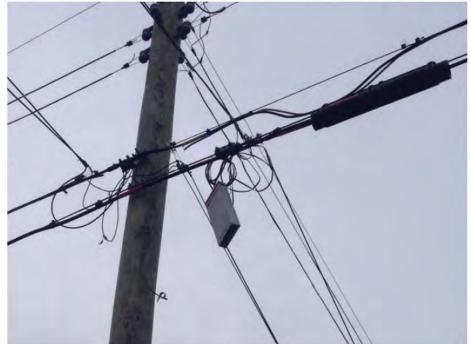
11. This photo from Sandpit Road, Bedford, IN, shows improperly secured cables. The cables are tied to the utility pole with rope (yellow arrow), which will eventually deteriorate, leaving the cables unsecured. The wind blows the unsecured cables, damaging the copper inside the wire and causing service issues.
