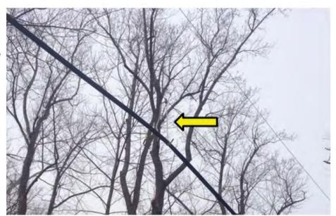
9. This photo from Maple Avenue, Noblesville, IN, shows a double-pole. The old pole (left) has only AT&T equipment attached to it. AT&T has not moved its facilities to the new utility pole. As a result, AT&T's equipment remains connected to an old, deteriorating pole, causing potential service and safety concerns.
