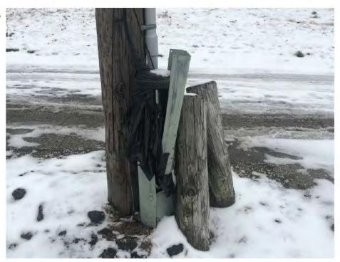
8. This photo from Town Hill Road, Nashville, IN, shows an improperly secured cable. Instead of being properly lashed, this cable is tied to a lash with a piece of rope (yellow arrow). The wind blows the unsecured service cables, damaging the copper inside the wire and causing service issues.
